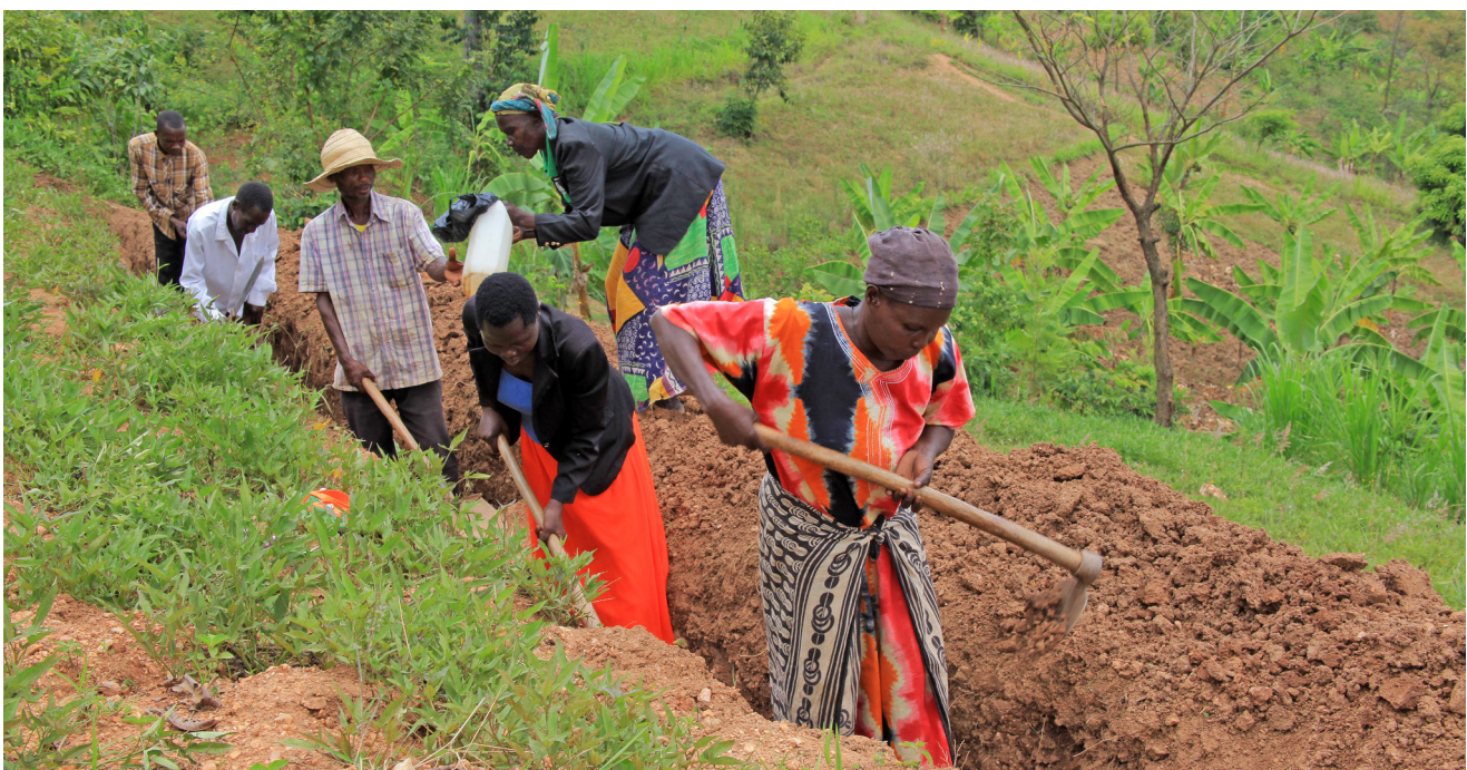
Digging contours in Bududa to reduce erosion and landslides
