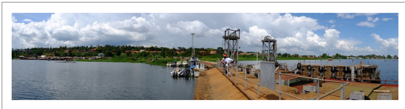
Figure 15: General view of Port Jinja
