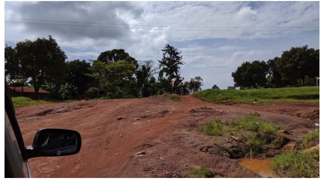
A damaged section of the access road to Kiyindi
