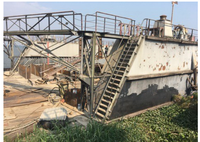
Dry port area
