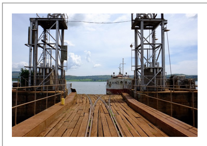
Figure 16: Pier at Jinja
