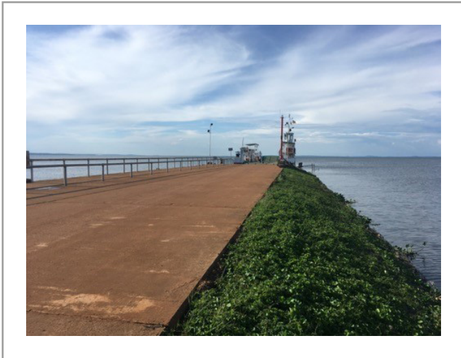
Figure 4: Good platform and landing facilities at Bugoma
