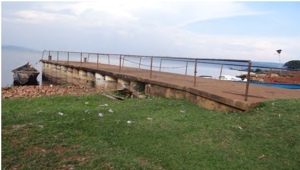
Figure 9. The original docking area for Kiyindi ferry – The exact spot for the envisioned development - (now abandoned because of low water levels)
