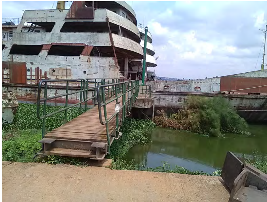
Figure 23. Abandoned ship and other infrastructure at Port Bell
