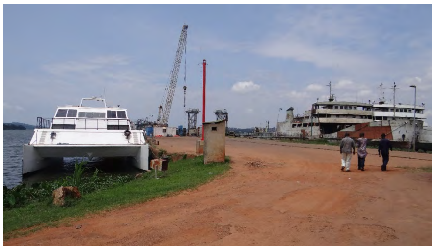
Figure 24. Road and parking yard conditions at Port Bell
