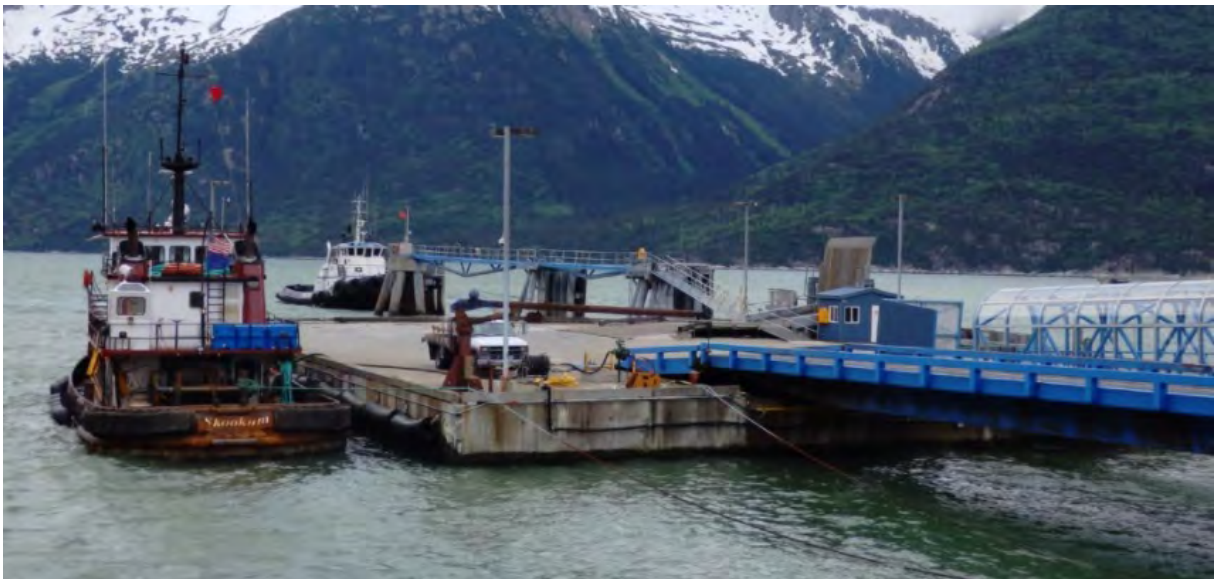
Figure 4.7 Floating Pier with Gangway
