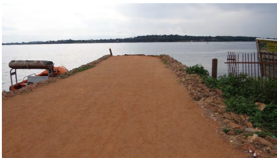
Figure 28. Existing pier area for Commercial ferry to Ssesse Islands at Nakiwogo Landing Site
