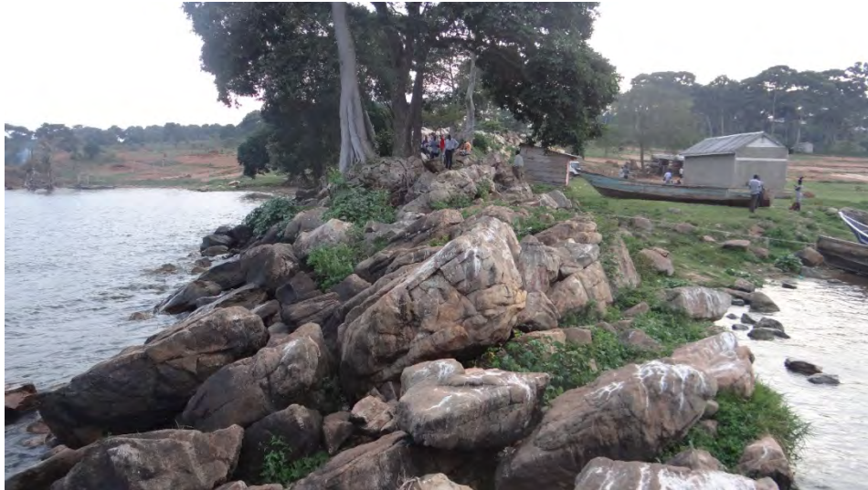
Figure 13. The proposed development site at Katosi Landing Site
