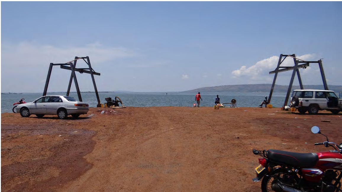
Figure 1. Proposed pier, car park and passenger waiting area at Masese Landing Site
