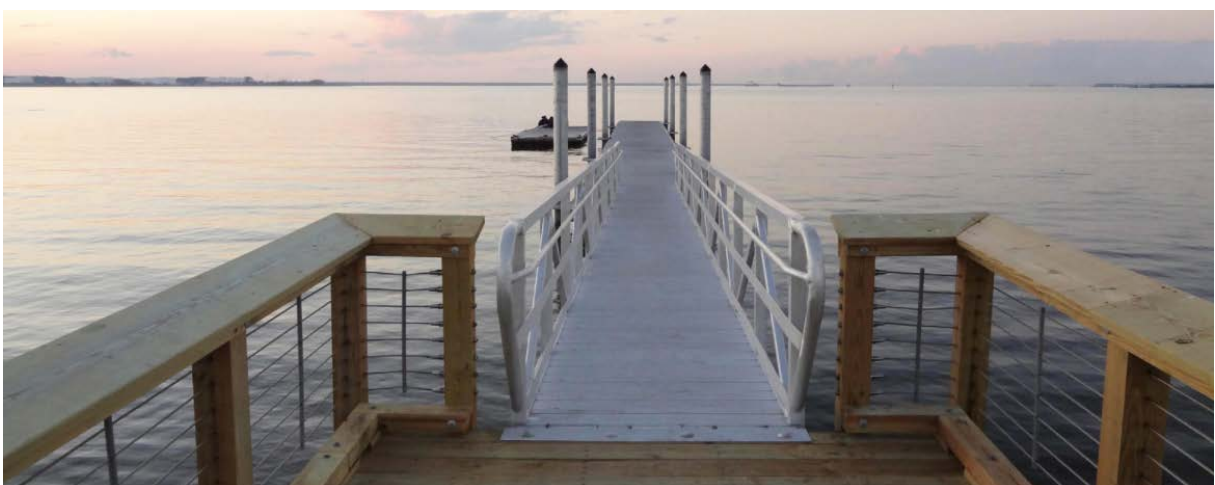
Figure 4.6 Gangway Connection
