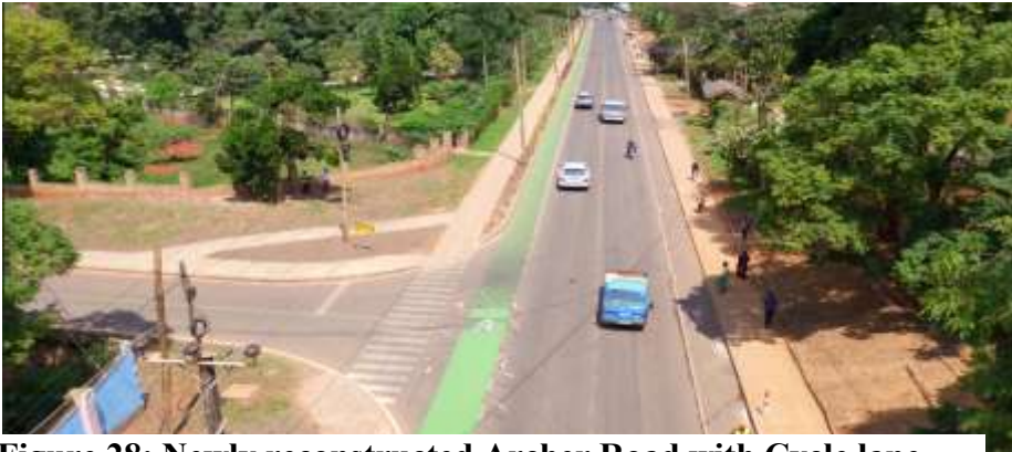
Figure 28: Newly reconstructed Archer Road with Cycle lane
