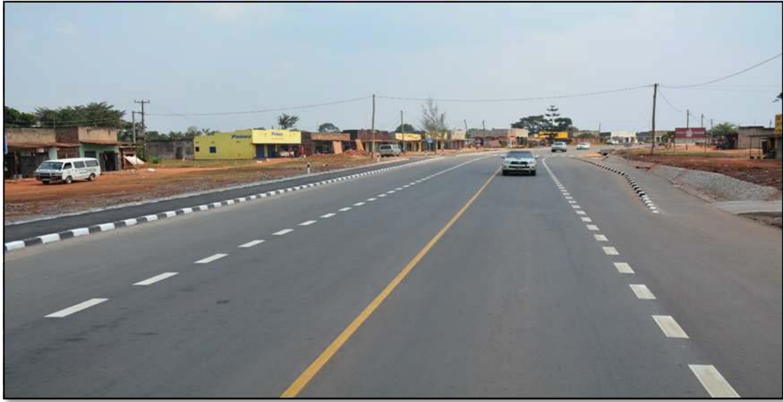
Figure 18: Completed Mukono-Kayunga-Njeru Road
