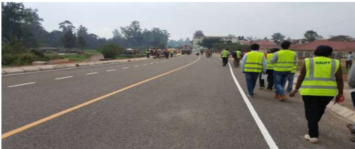
The completed Kamwenge-Fortportal Rd
