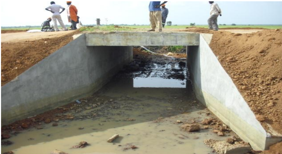
Completed Reinforced Concrete box culvert at Olyanai Swamp under Lot 3
