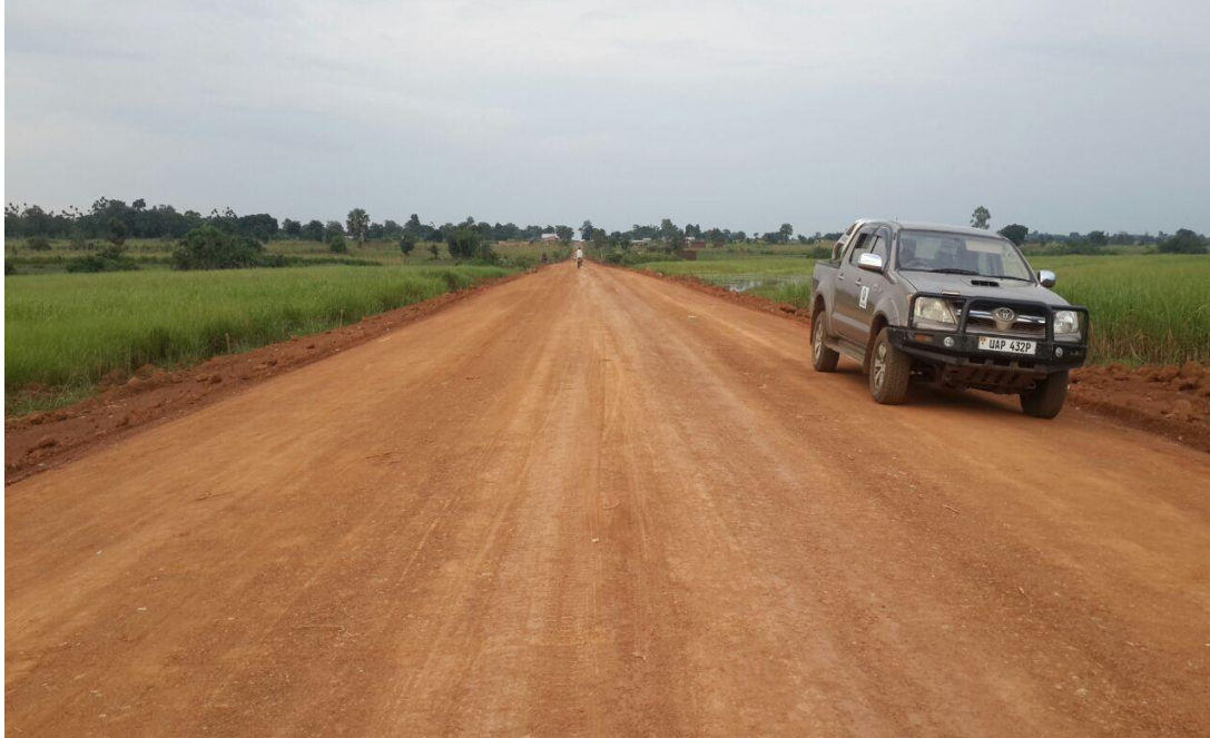
Completed G15 fill material at Abalang under Lot 1
