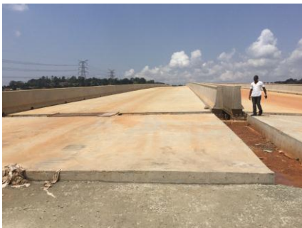
Construction of Kampala – Entebbe Express way - Nambigirwa Bridge
