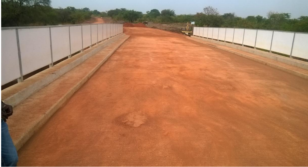
Completed Nyawa Bridge under Lot 2
