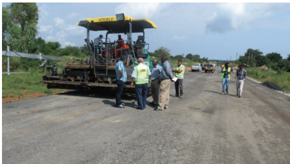
Figure 7. 1: Showing Upgrading Gravel Roads
